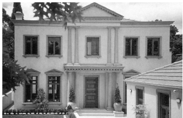
Figure 9.3 Decorative External Façade Mouldings. Image supplied by www.unitex.com.au .
